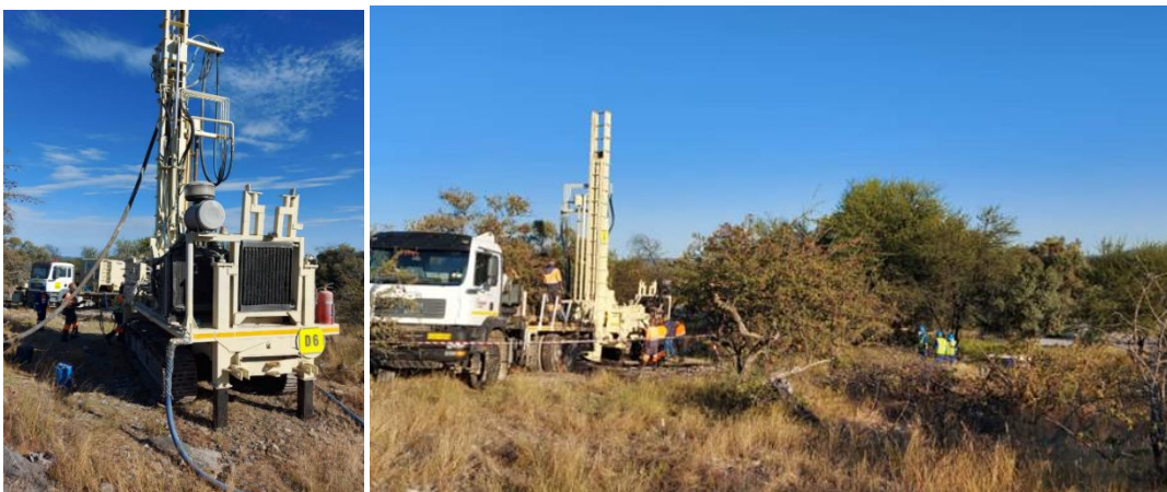
Figure 1: Reverse circulation drill rig in operation at Khusib Springs
